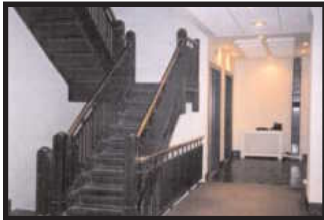
Original slate stairs and brass railings.
