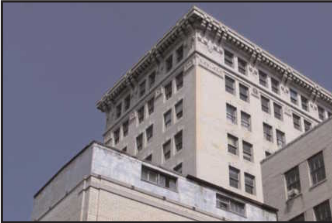
An indoor squash court may be seen atop the addition's rear second floor.
