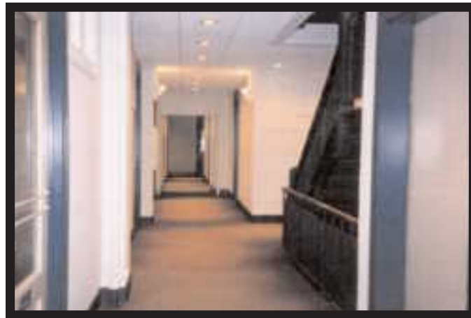
A remodeled hallway with drop ceiling.
